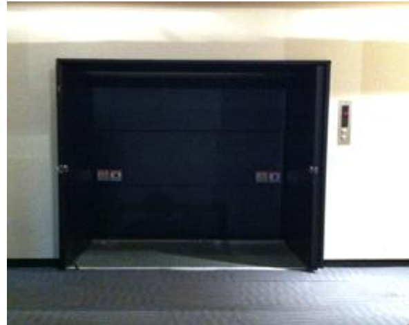
The inner door (B3 floor)
